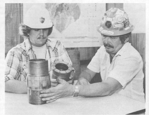
DIAMOND-IMPREGNATED CORING BIT is held by LANL's Jamie Gardner (left), one of the two principal investigators on the Valles Caldera project (the other is Jeff Hulen of the University of Utah Research Institute). At right is Ron Jacobson (6252) with a reamer shell that brings the corehole into final gage.
